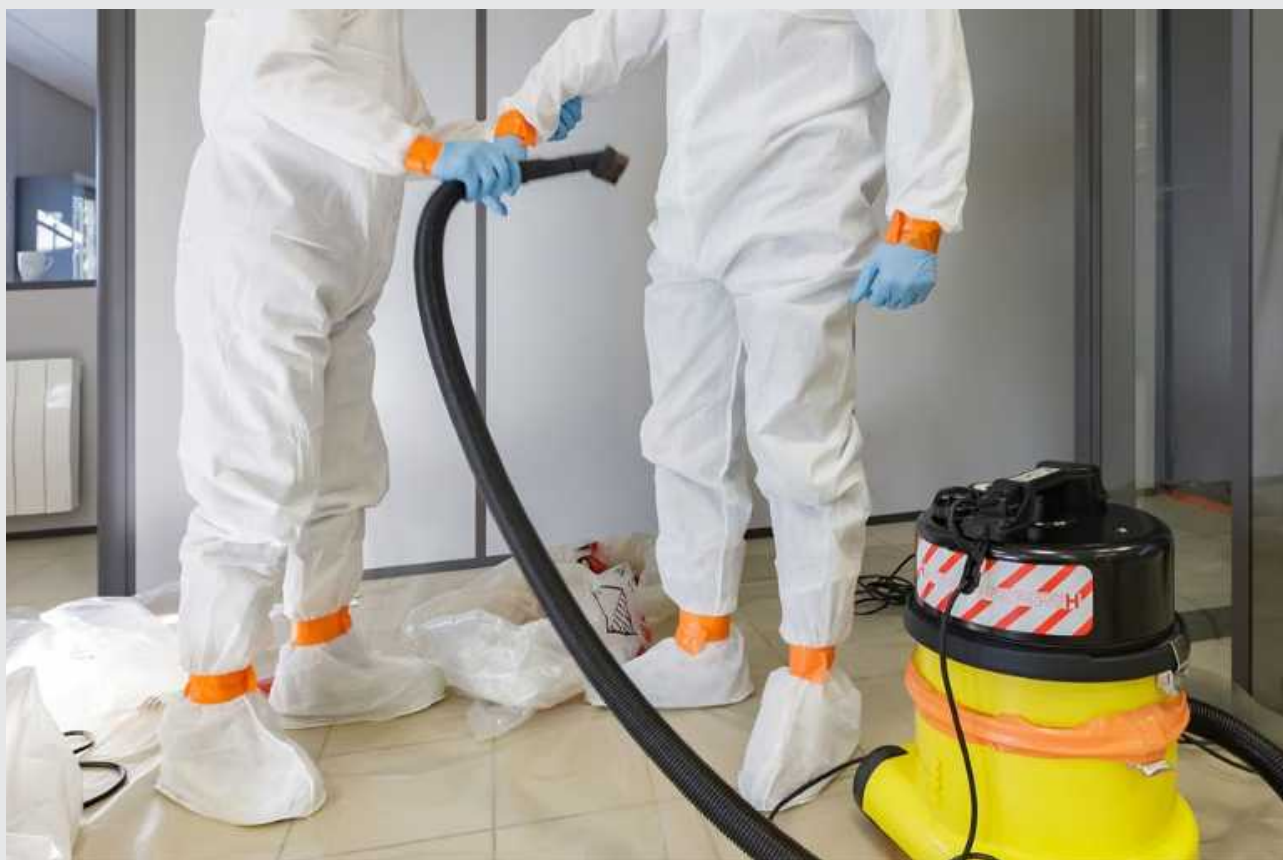
Figure 8-6: Example of cleaning using a vacuum cleaner
