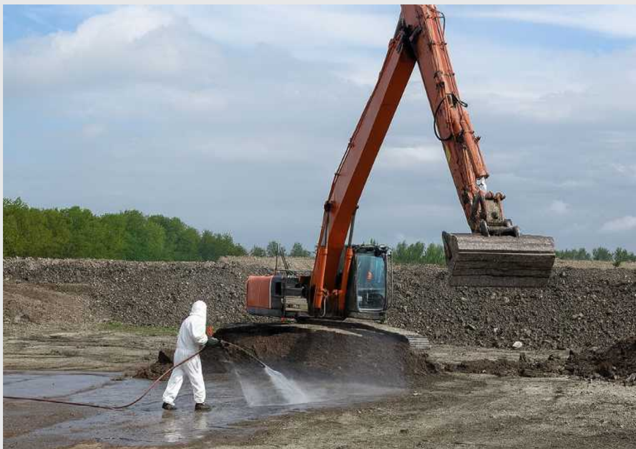
Figure 12-2: Wetting of WCA to prevent dust
