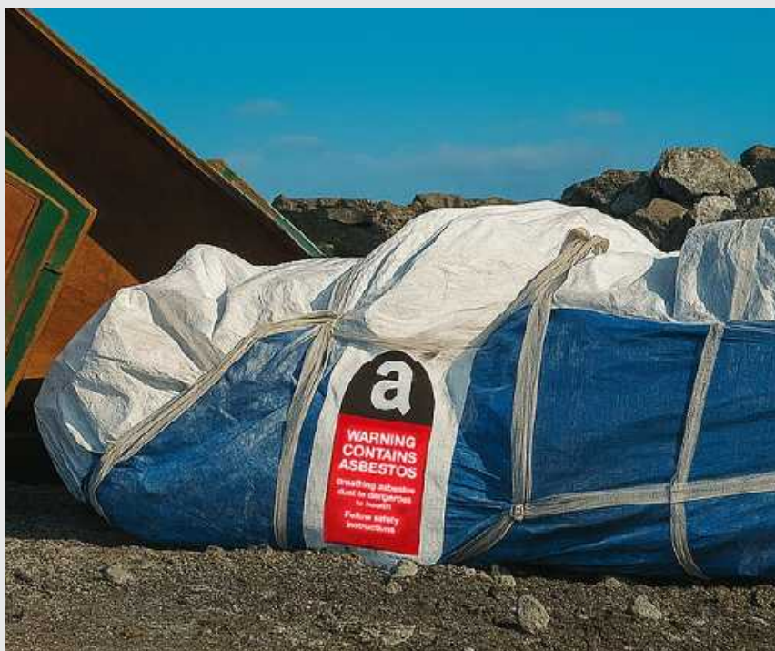
Figure 12-3: WCA disposed in sealed bags
