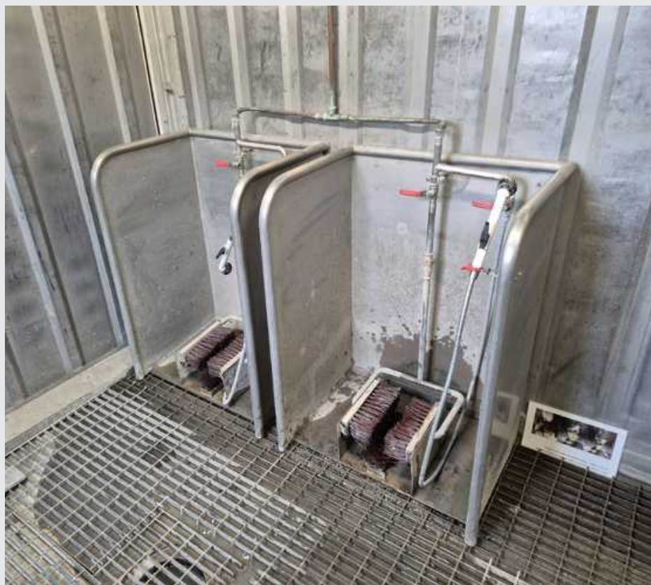
Figure 15-3: Footwear washing facilities inside a decontamination chamber
