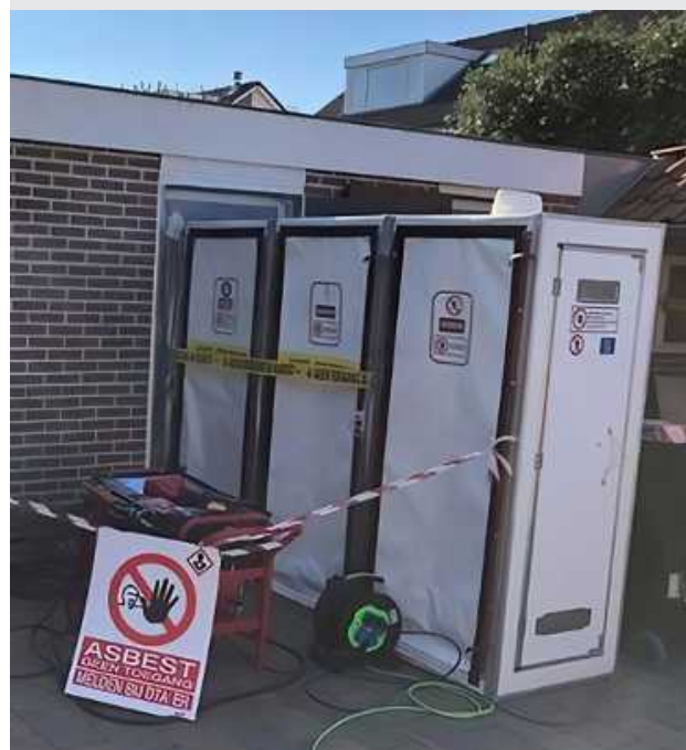
Figure 8-5: Example of a decontamination unit set-up
