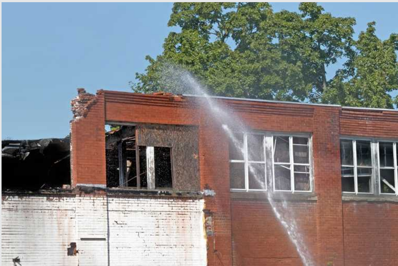
Figure 8-1: Example of wetting a building containing asbestos
