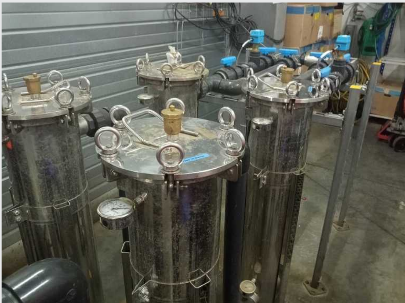
Figure 14-9: Filters to remove asbestos fibres from waste water at a train dismantling facility in France
