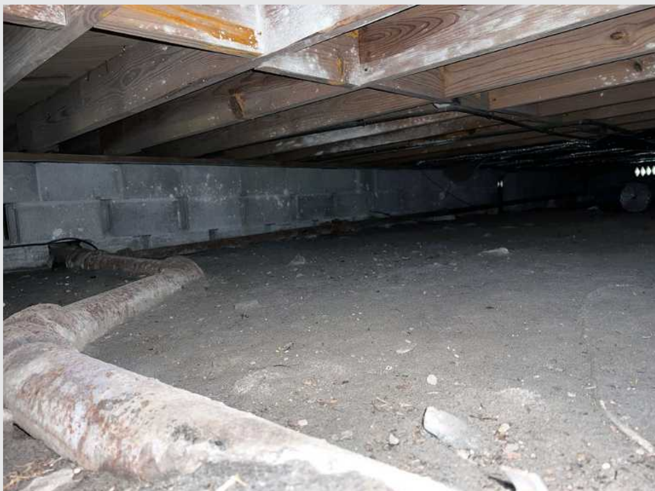
Figure 13-3: Work in crawl spaces
