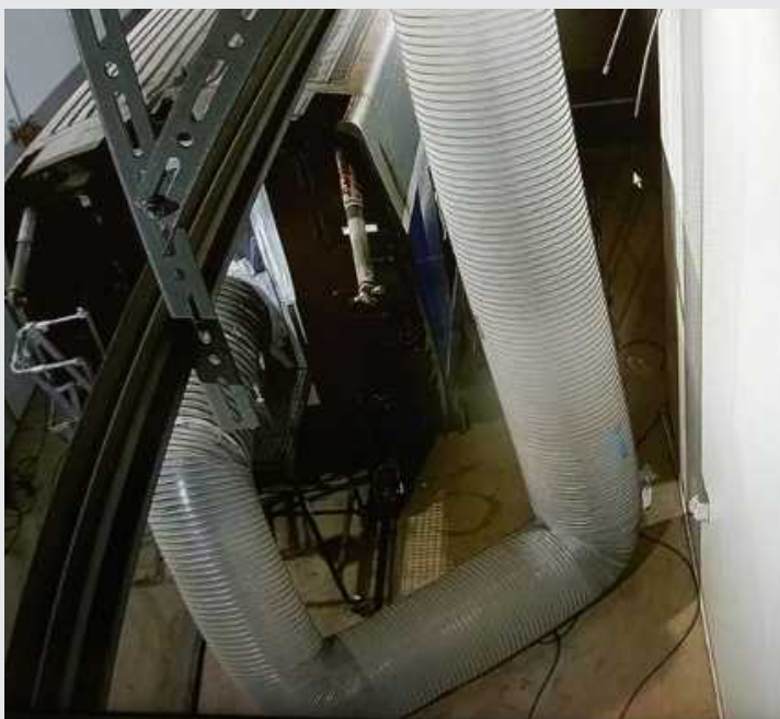
Figure 14-8: Air extraction system used during the removal of asbestos coatings by abrasive blasting from a train carriage at a train dismantling facility in France
