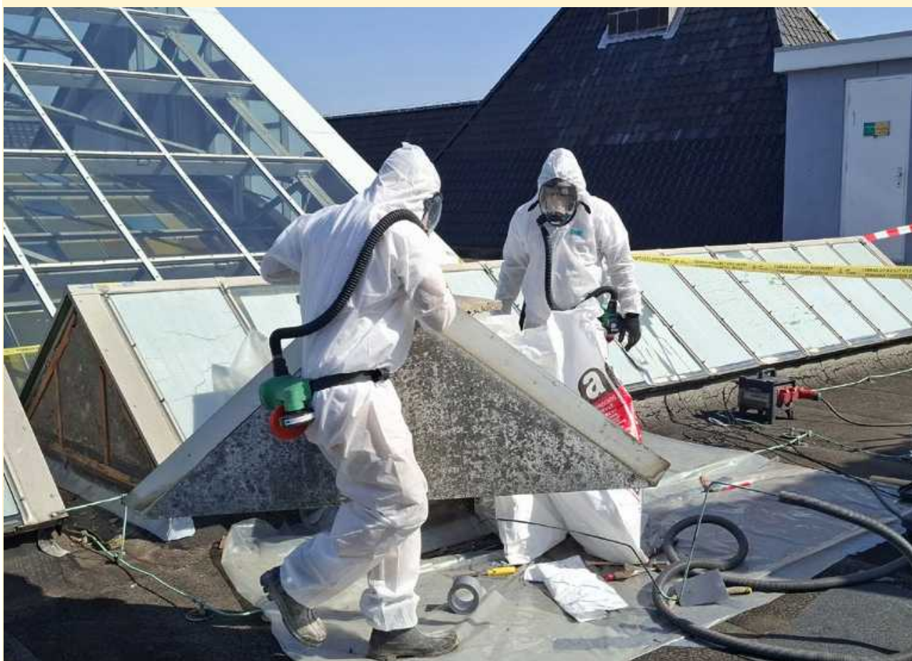
Figure 4-4: Workers removing asbestos plates on the roof
